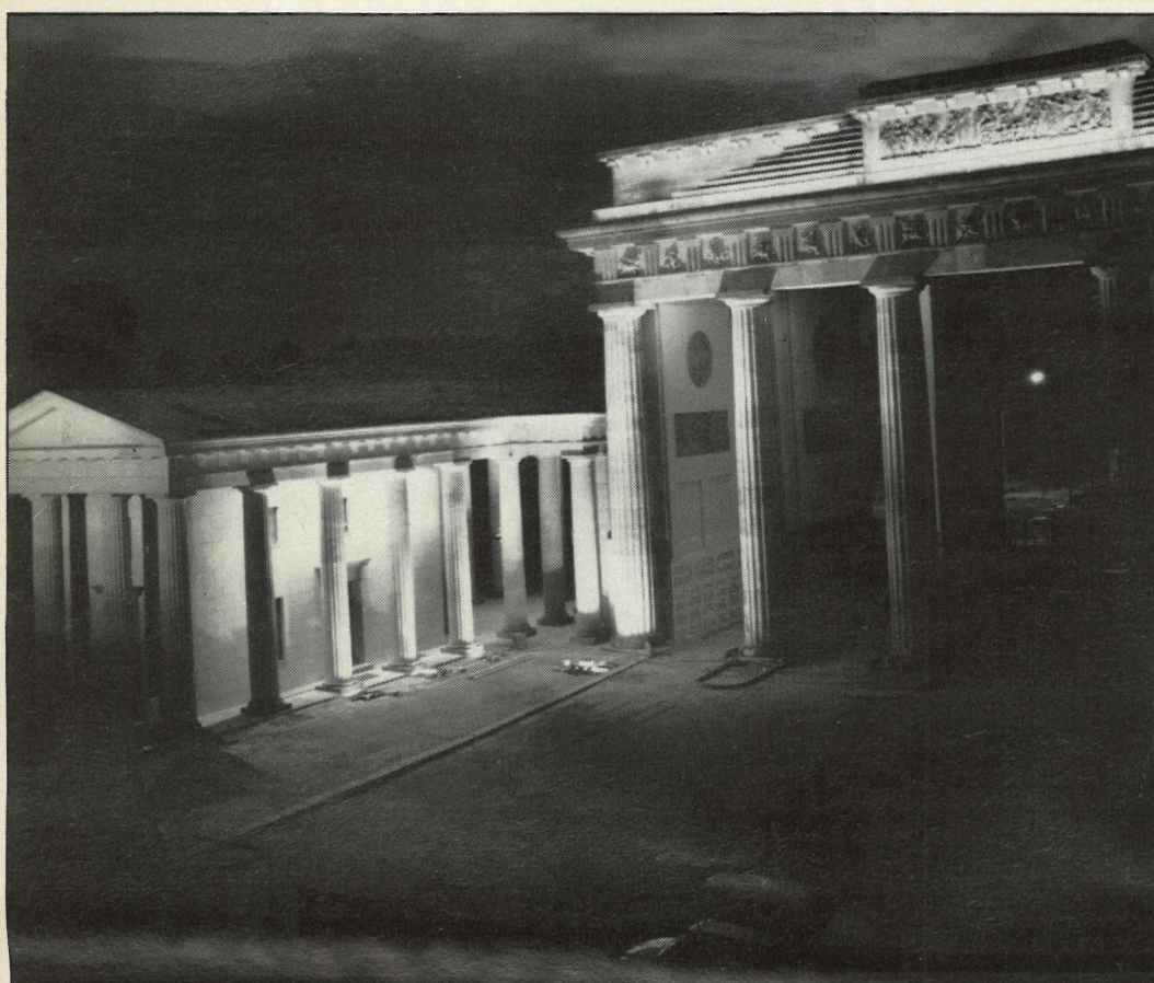
Testing the new floodlighting scheme for the Brandenburg Gate, Berlin's famous landmark (left). Fluorescent lighting being installed at the upper level to light the building above the cornice (right).
